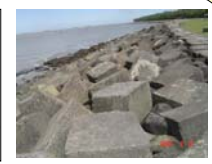
Fig. 6: Bank protection works, Chittagong
