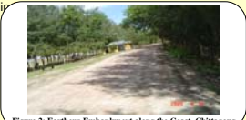
Figure 2: Earthen Embankment along the Coast, Chittagong
