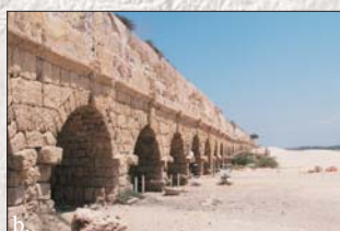
The north-south aqueduct bringing water to Caesarea, dated to the first few centuries AD, strengthens our conclusion of absence of vertical tectonic movements over the last 2,000 years.
